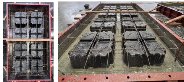
(a) Before casting
