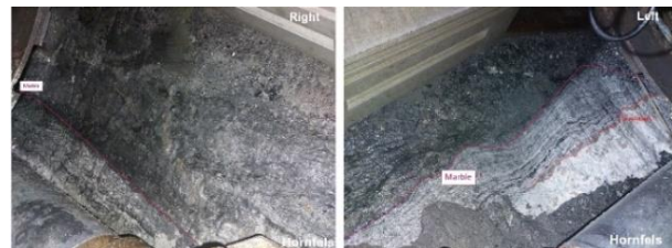
Fig. 6 Geological images after excavation on Head Cutter to tail shield gap Ring Nos. 4363, 4364, 4367
