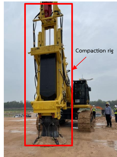
Fig.4 The RIC compaction rig mounted on excavator.
