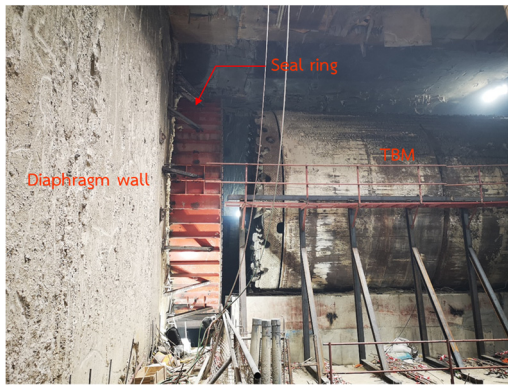
Figure 11 Preparation for TBM launching work
