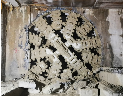
Figure 14 TBM break-in during the construction of MRT Orange Line Project
