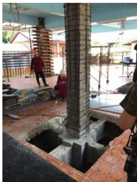
Fig. 5 Concrete jacketing details.
