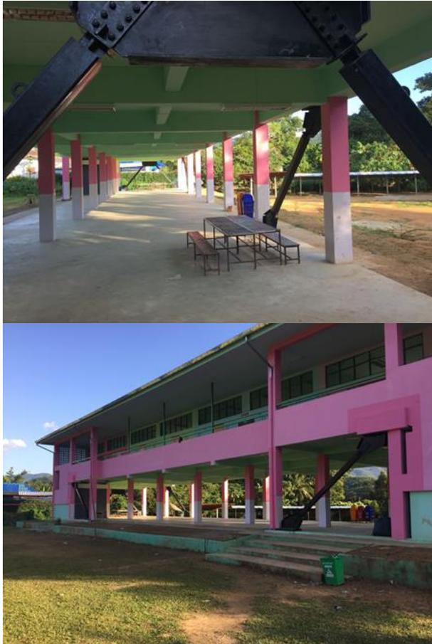
Fig. 4 BRB configuration of the prototype building.
