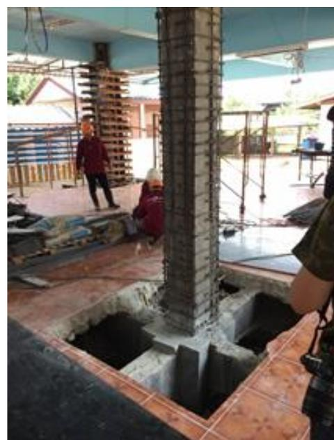
Fig. 5 Concrete jacketing details.
