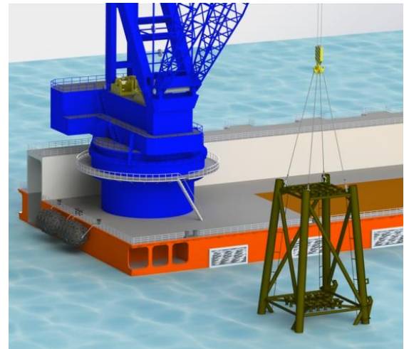
Figure 11: Revolve crane to starboard to lower jacket
